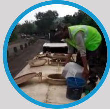
Addition of Liquid Chemical Additive
