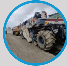
Pulverization of soil with Recycler
