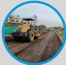
Compaction by Soil Compactor
