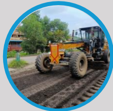
Grading & Profiling with motor Grader
