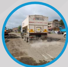
Cement Spreading by Microprocess or Controlled Spreader Truck
