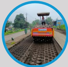
Compaction by Pad Foot Roller
