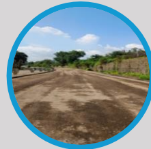
Final surface after Compaction
